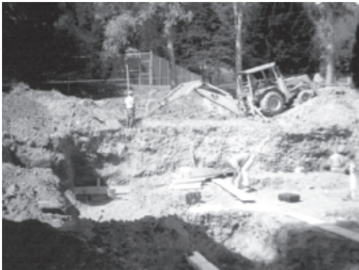
All Saints Chapel Construction Site
